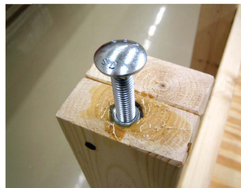
Here we just drilled the hole for the shank of our 1/2-inch carriage bolt. Then drilled a shoulder for the nut. You'll need to use a chisel to conform the hole to the nut and press fit it in. We added a little 5-minute epoxy to keep the nut in place.
